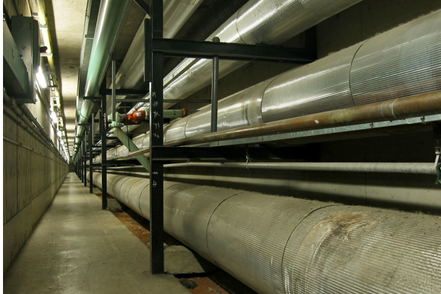
Figure A.1.2 Steam Pipes
