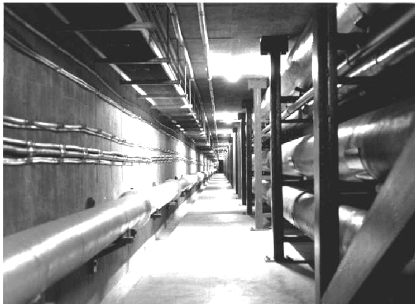
Figure A.1.3 Utilities housed within University of Toronto Utility Tunnel
